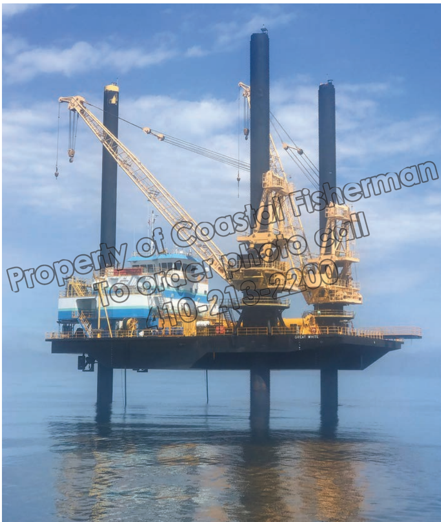
In advance of the US Wind offshore wind farm project, a 330-foot meteorological tower is being constructed 18-miles off the coast of Ocean City. The tower, sunk in 88-feet of water, will be used to collect wind resource data in advance of the controversial installation of offshore wind turbines.
